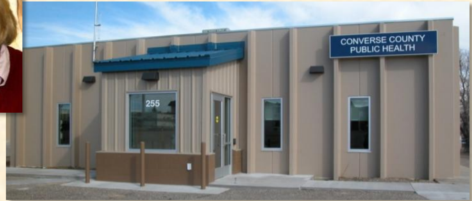
Converse County Public Health moved into their new building in 2010.
